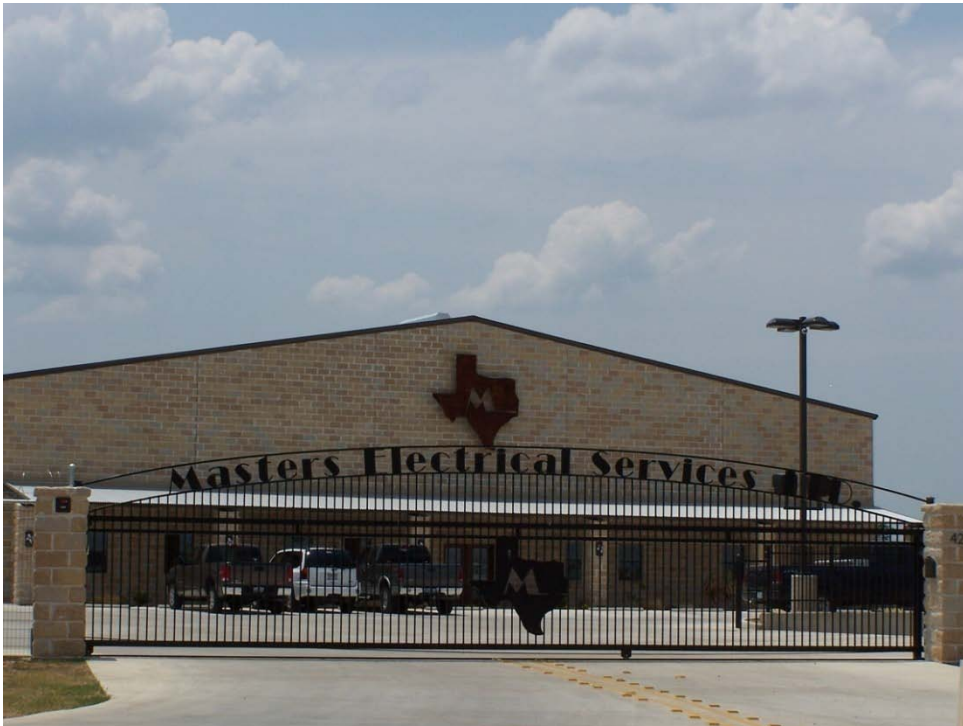
MASTERS ELECTRICAL SERVICES LTD. 4239 W. IH-10 :: SEGUIN, TEXAS 78155
